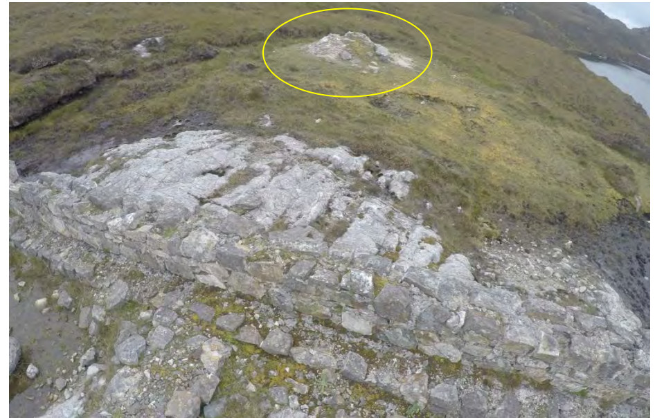
BNC 2: SW footings looking SW towards lime clamp (highlighted)
