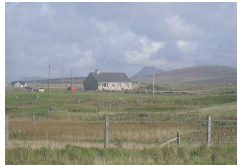
Fig 36: A cavity blockwork croft house from the late 1960s
