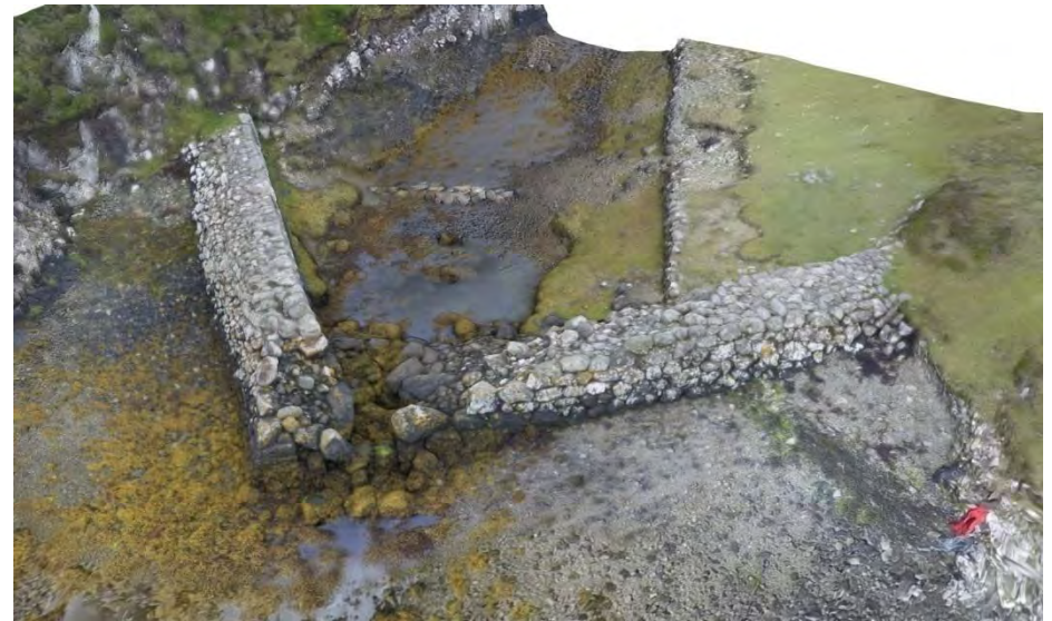
BNC 3: aerial view of dam from NE
