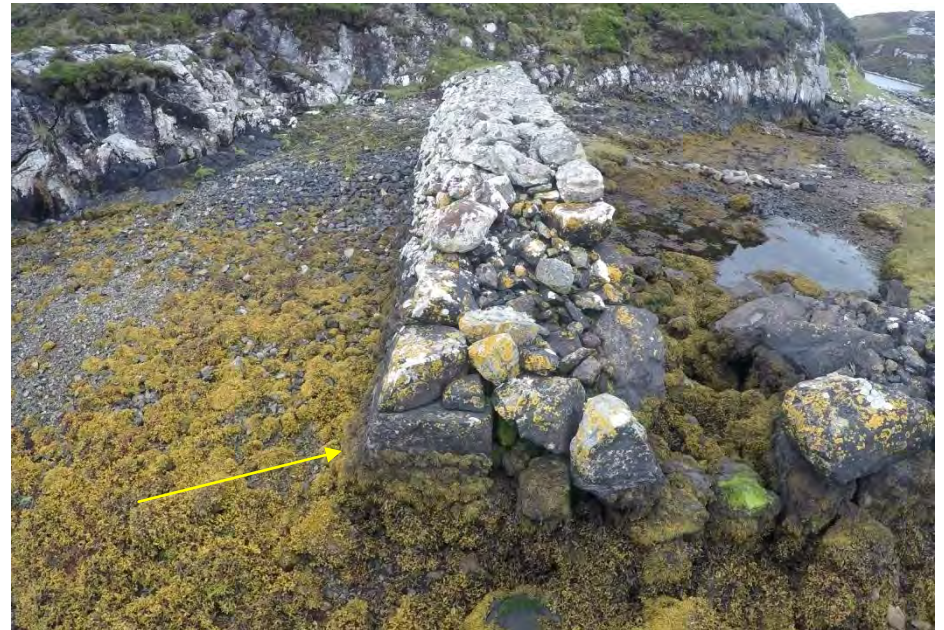
BNC 3: dam looking SW from centre, quoin stone highlighted
