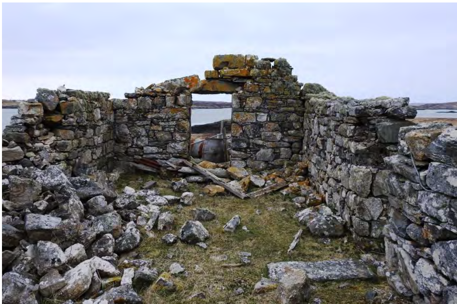
Fig 57: BM 4 interior looking west
