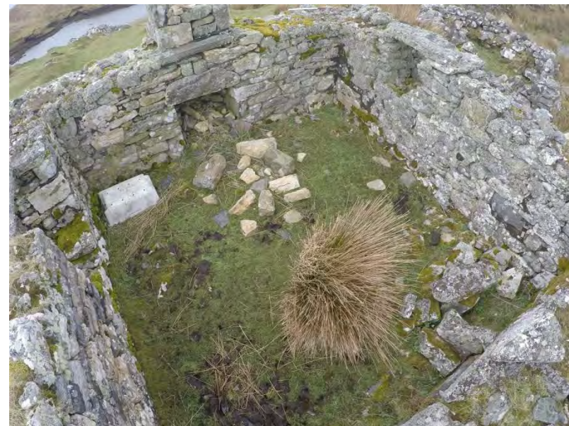
Fig 59: BM 8 interior view looking north-west
